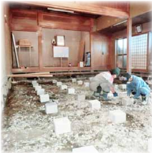
Ishinomaki worship hall damage
