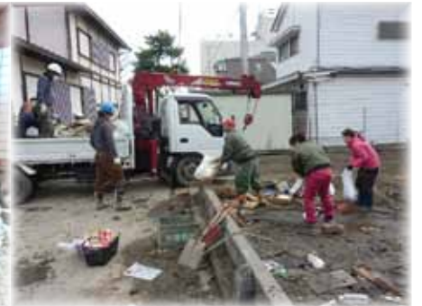
Clearing the debris
